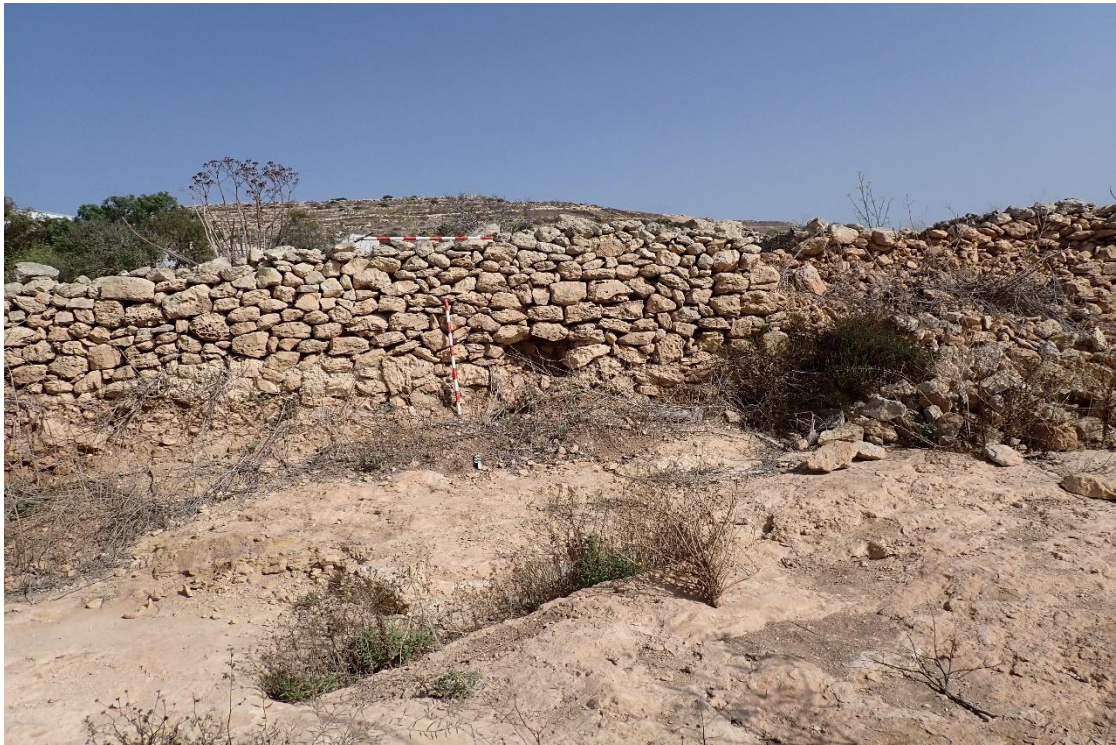
FIGURE 26: EXPOSED AGRICULTURAL TRENCH AND CONTINUATION OF CENTRAL RUBBLE BOUNDARY WALL, LOOKING NORTH
