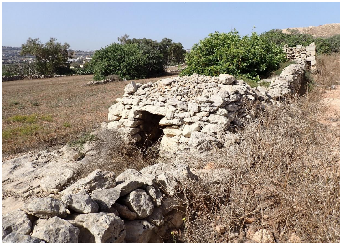
FIGURE 37: STONE HUT (GIRNA) ON SOUTHERN SIDE OF RUBBLE BOUNDARY WALL, LOOKING S-WEST
