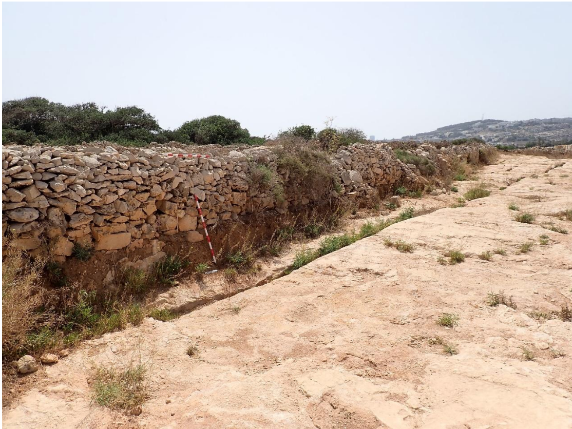
FIGURE 60: RUBBLE BOUNDARY WALL IN THE CENTRAL-NORTH AREA, LOOKING S-EAST
