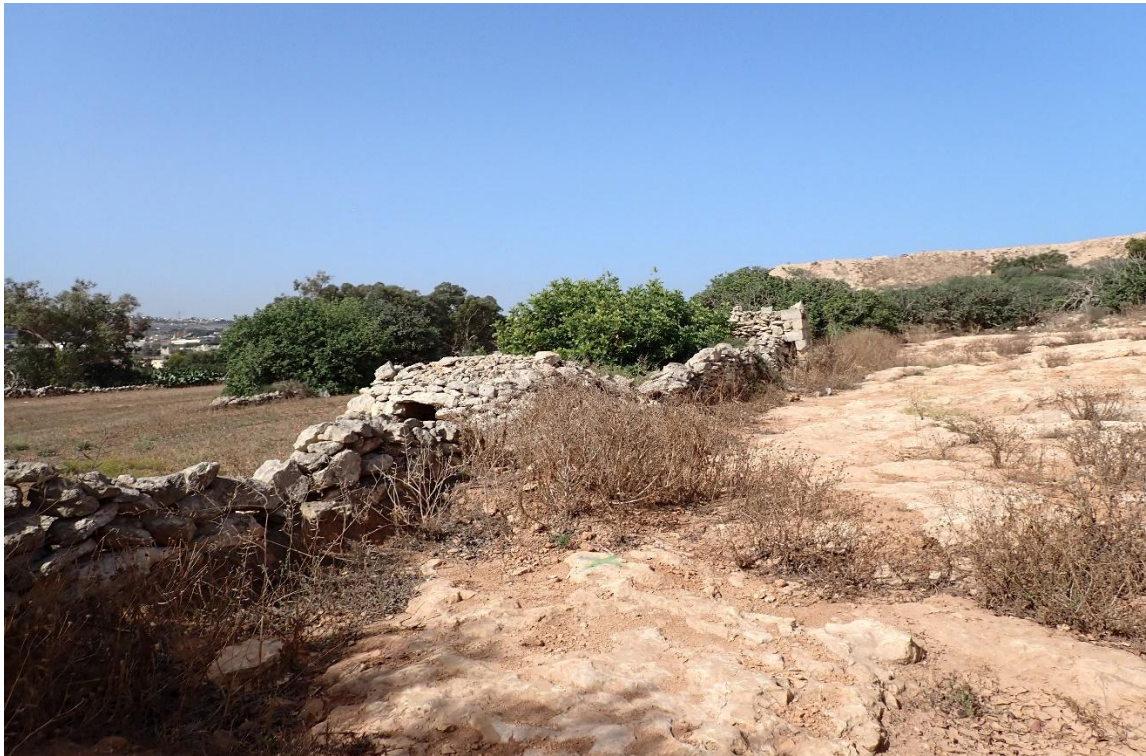
FIGURE 36: SOUTHERN RUBBLE BOUNDARY WALL WITH STONE HUT (GIRNA), LOOKING S-WEST
