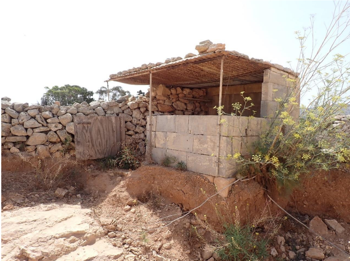
FIGURE 48: MODERN HAUNTING POST IN THE EASTERN PART OF SITE, LOOKING EAST
