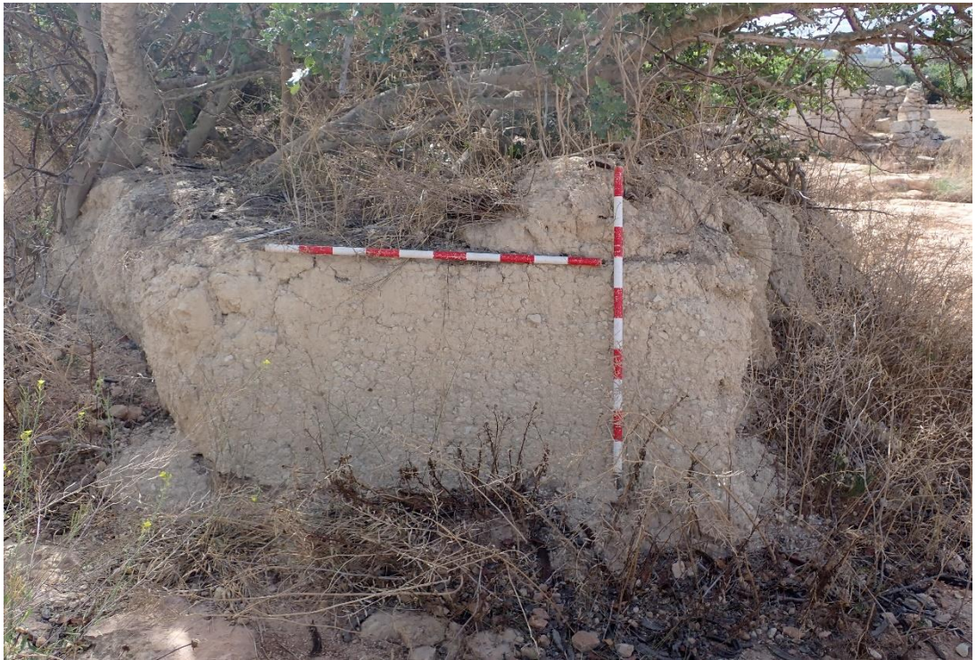
FIGURE 20: NORTH FACING SECTION OF ORIGINAL SOIL WITH NO INCLUSIONS, LOOKING SOUTH
