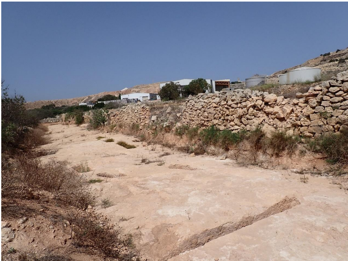
FIGURE 55: NORTHERN RUBBLE BOUNDARY WALL, LOOKING N-WEST
