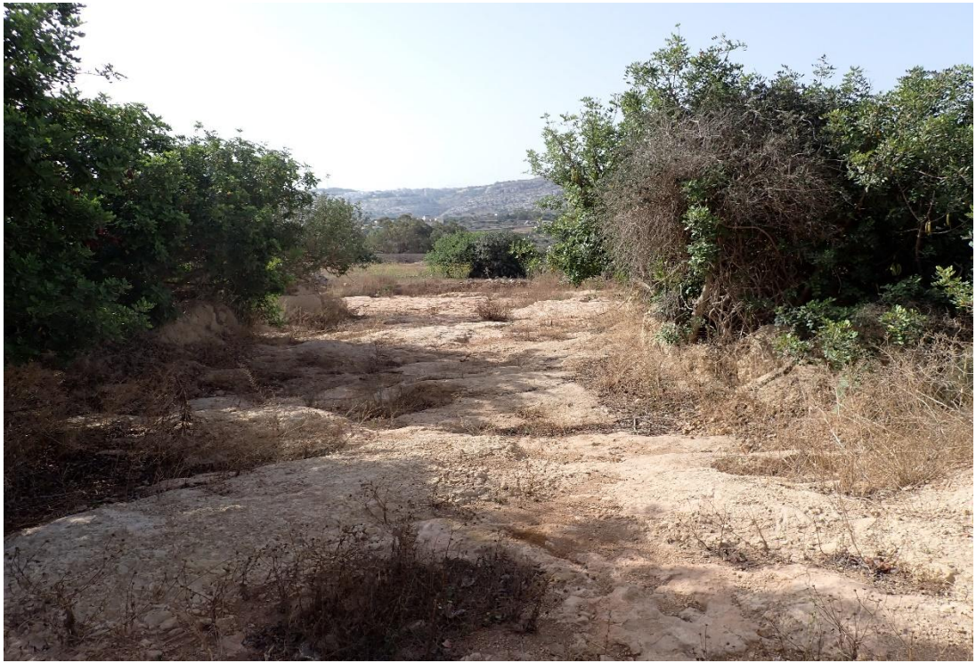
FIGURE 12: WESTERN AREA STRIPPED OF SOIL, LOOKING SOUTH
