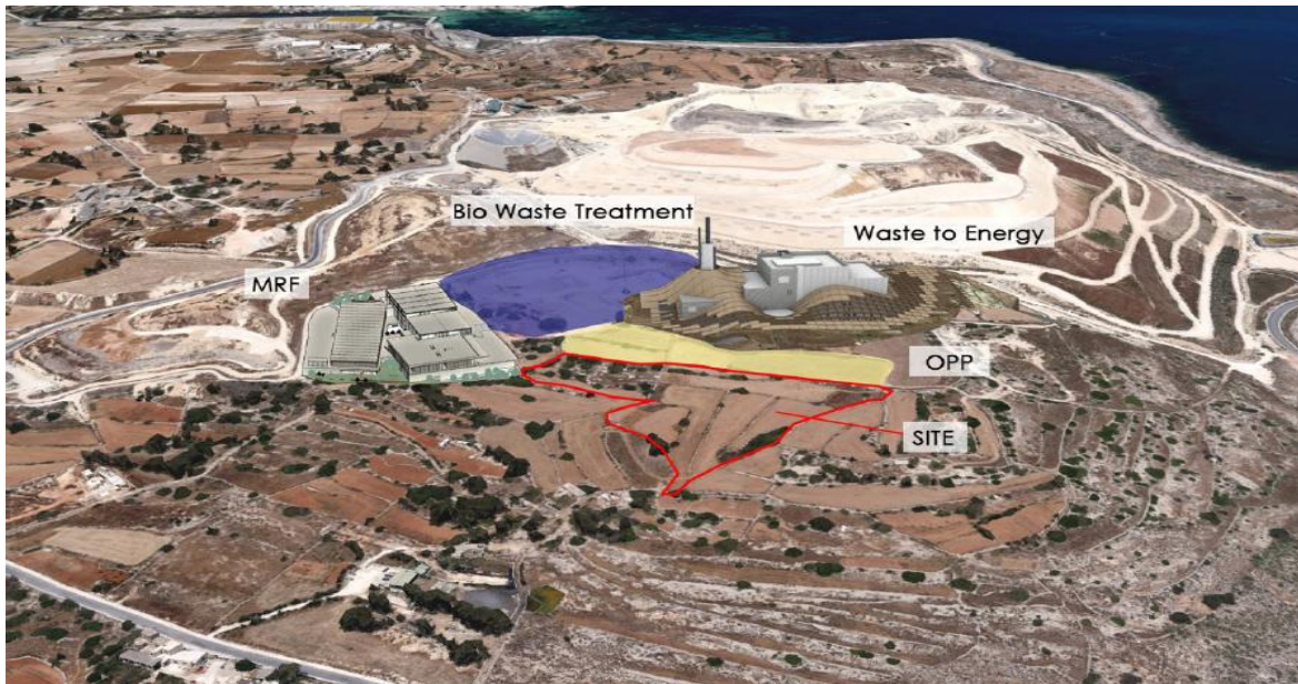
Figure 2: Site location (Source DESIGN report)
