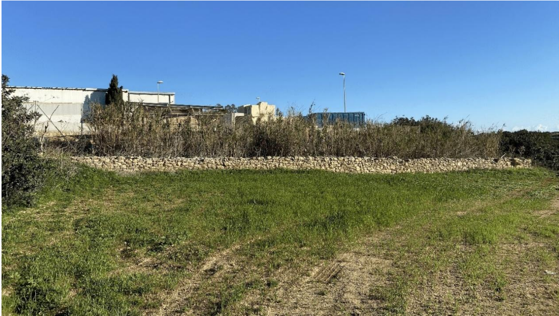
FIGURE 17: NARROW STRIP OF LAND SURROUNDING THE EXISTING BIODIGESTER PLANT DOMINATED BY THE INVASIVE ARUNDO DONAX
