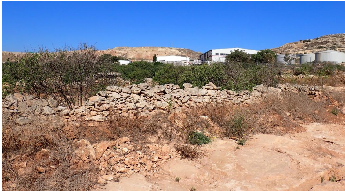
FIGURE 24: EXAMPLE OF RUBBLE WALLS WITHIN THE AOI (PHOTO TAKEN JULY 2024)
