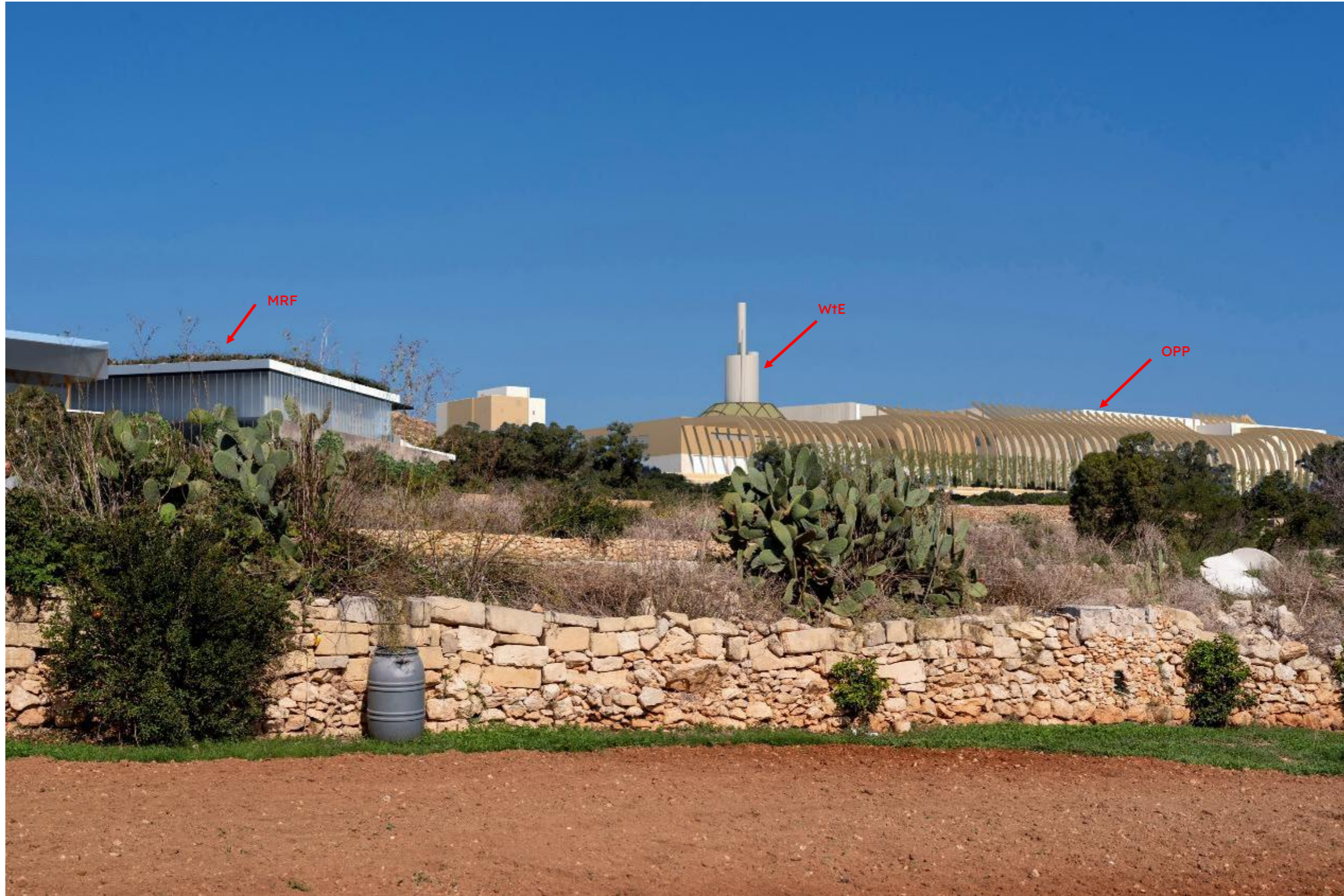
FIGURE 29: CUMULATIVE VIEW SHOWING PHOTOMONTAGE OF THE MRF, WtE AND OPP PLANT ONLY AT VIEWPOINT4 4
