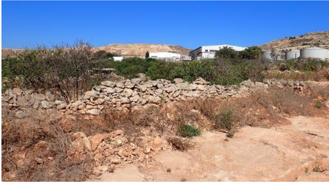
FIGURE 25: EXAMPLE OF RUBBLE WALLS WITHIN THE AOI (PHOTO TAKEN JULY 2024)
