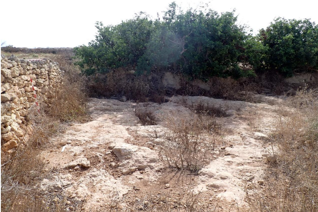
FIGURE 102: WESTERN ACCESS TO SITE. AREA STRIPPED OF SOIL WITH TWO AGRICULTURAL TRENCHES EXPOSED. LOOKING EAST
