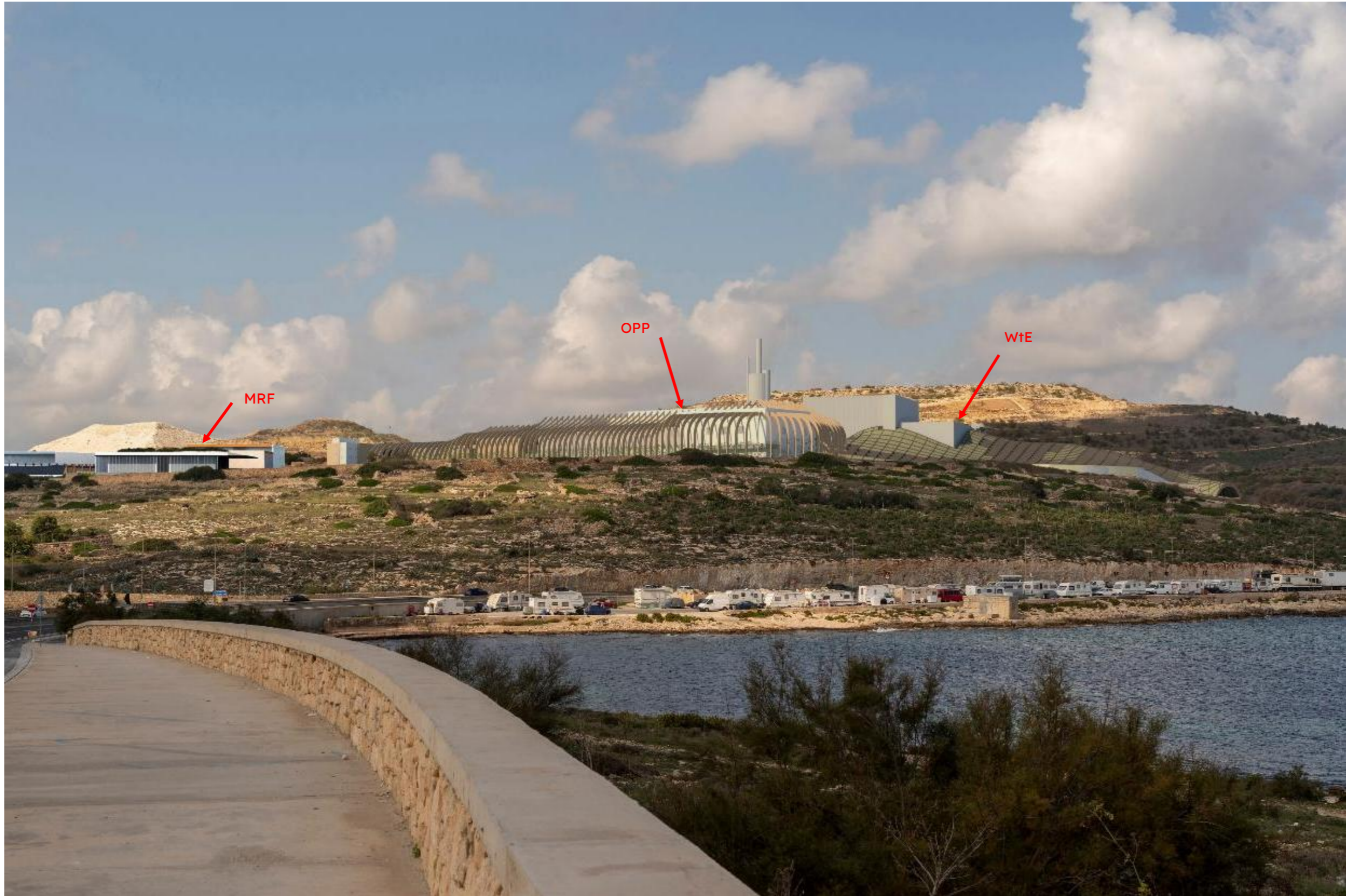
FIGURE 56: CUMULATIVE VIEW SHOWING PHOTOMONTAGE OF THE MRF, WtE AND OPP PLANT ONLY AT VIEWPOINT5
