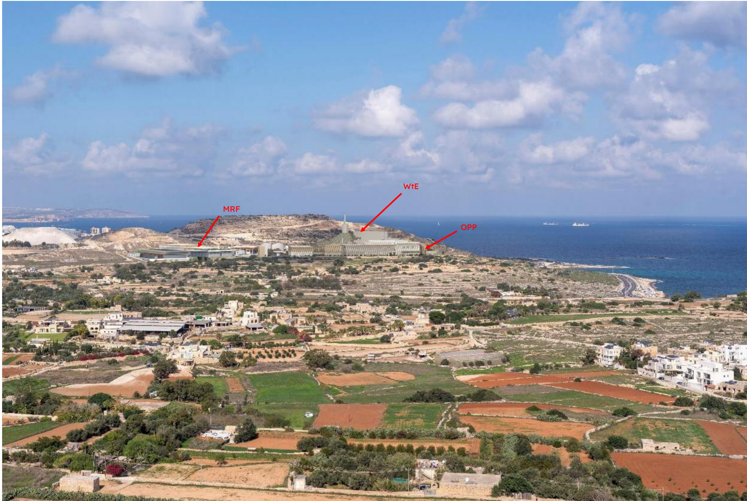
FIGURE 62: CUMULATIVE VIEW SHOWING PHOTOMONTAGE OF THE MRF, WtE AND OPP PLANT ONLY AT VIEWPOINT 7
