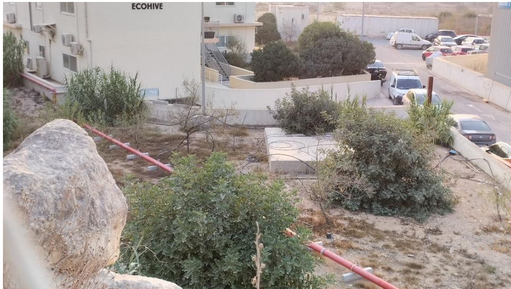
FIGURE 33: LANDSCAPED AREA AROUND THE EXISTING ANAEROBIC DIGESTER PLANT
