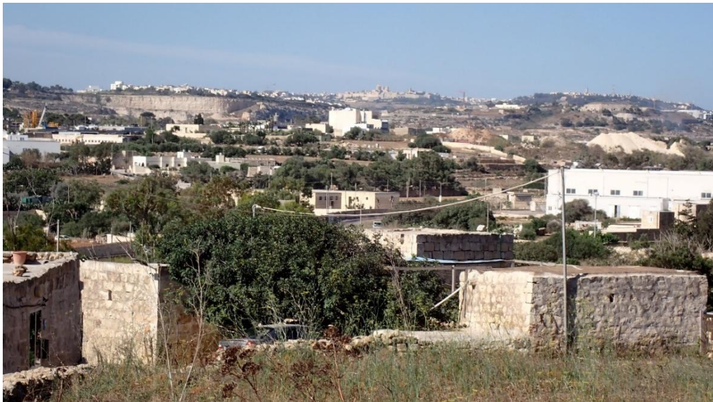
FIGURE 38: FARMHOUSES TO THE SOUTH-EAST OF THE PROPOSED SITE
