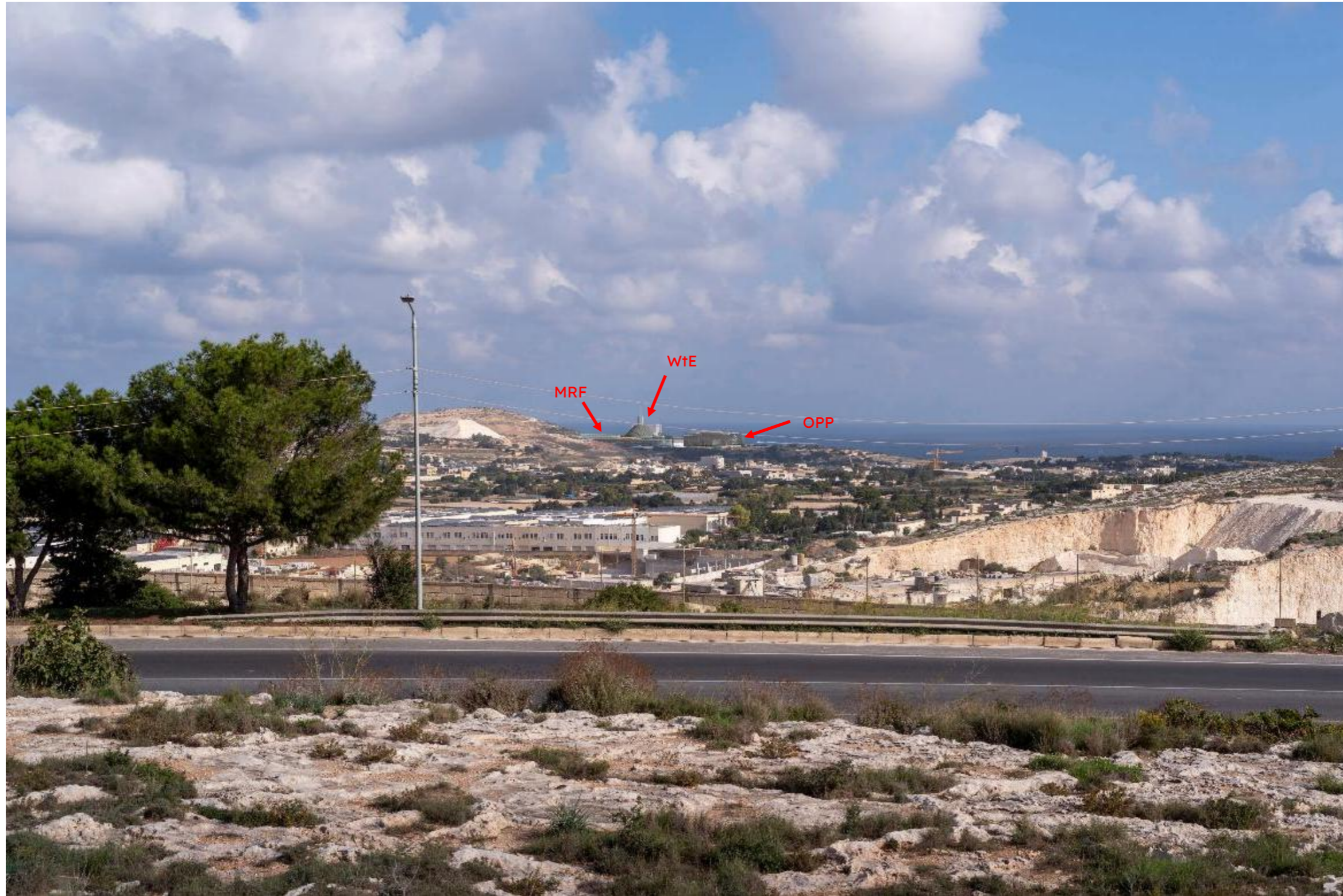
FIGURE 44: CUMULATIVE VIEW SHOWING PHOTOMONTAGE OF MRF, WtE AND OPP PLANT ONLY AT VIEWPOINT 1
