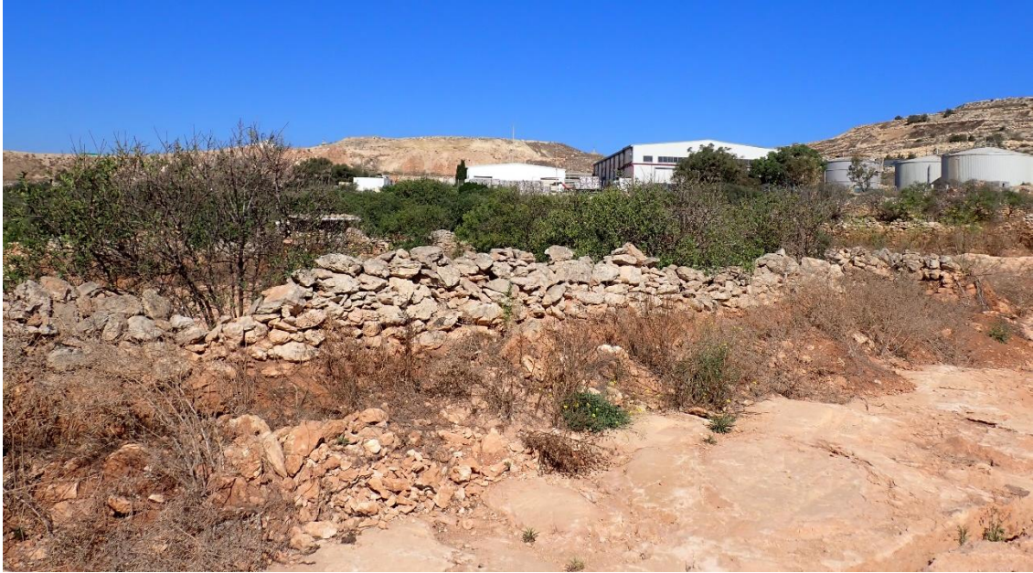
FIGURE 81: RUBBLE WALLS WITHIN THE AOI (PHOTO TAKEN JULY 2024)
