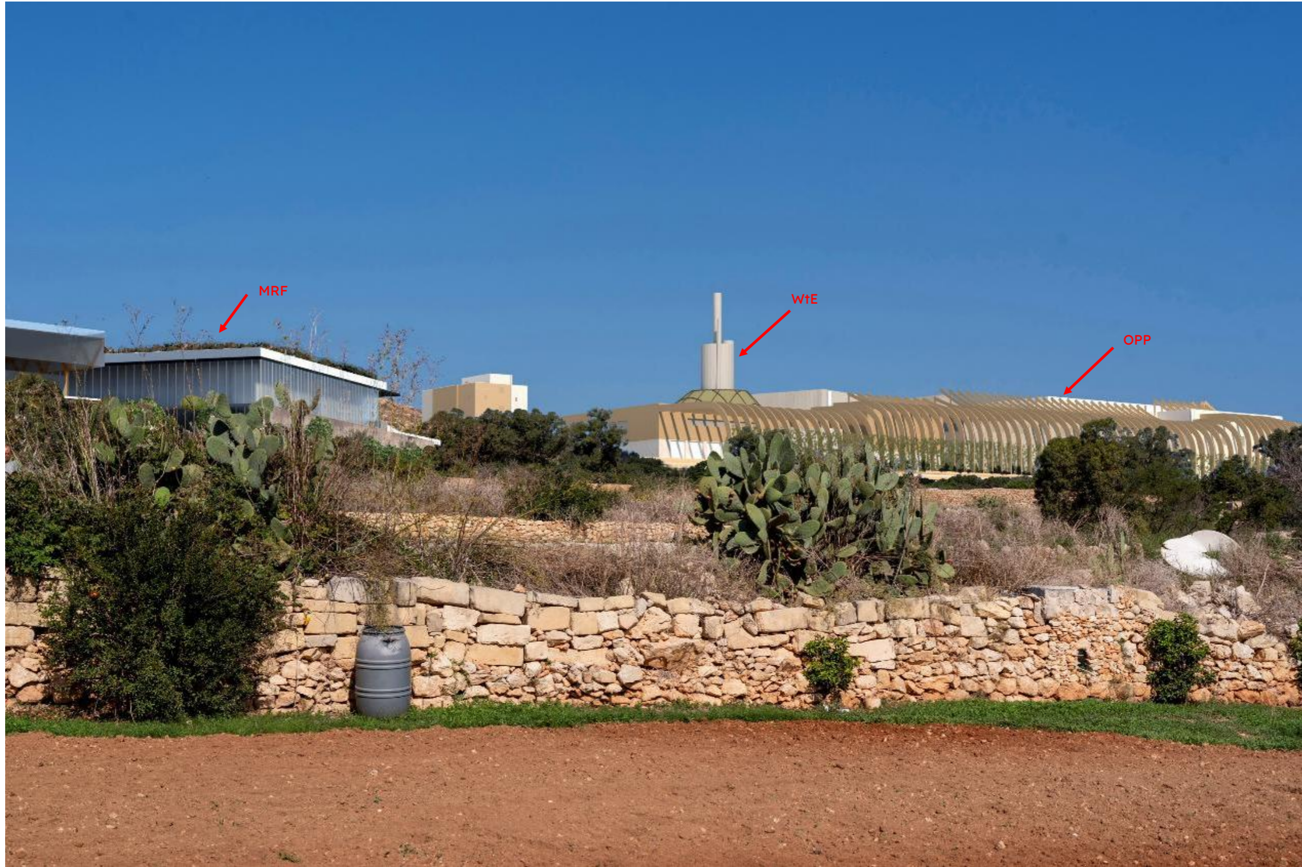
FIGURE 53: CUMULATIVE VIEW SHOWING PHOTOMONTAGE OF THE MRF, WtE AND OPP PLANT ONLY AT VIEWPOINT4
